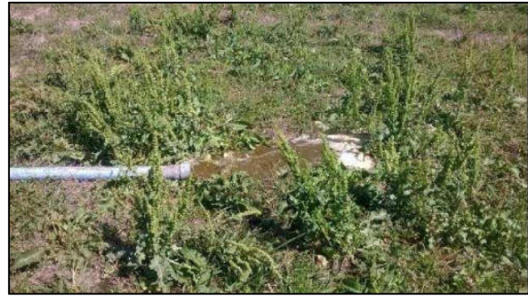
Figures 2-7 Left: A polishing pond in a WSP system. Right: Direct discharge on terrain; from (Houlbrooke, 2015)
