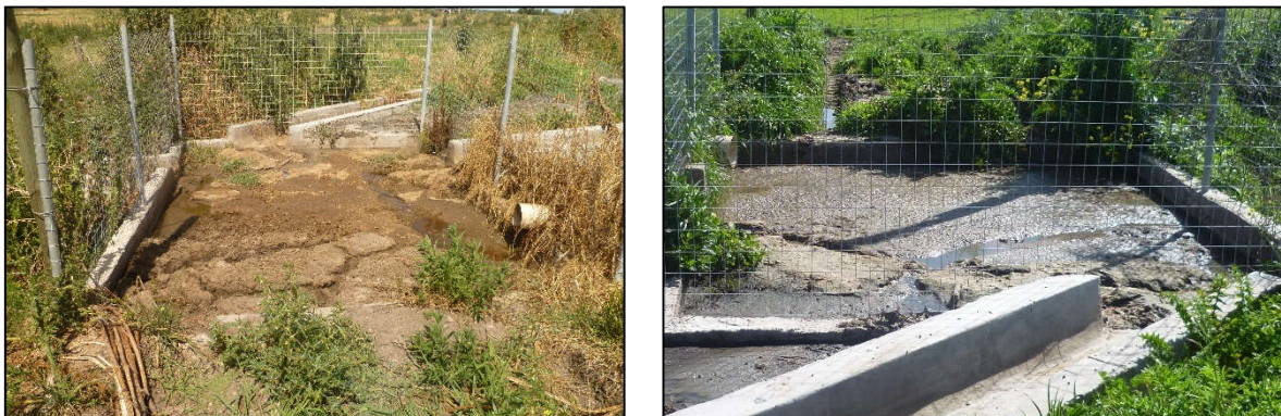
Figures 5-1 Solids chamber on 14/12/2016 (left) and 21/09/2016 (right)
