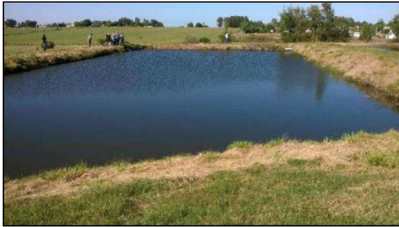
Figures 2-7 Left: A polishing pond in a WSP system. Right: Direct discharge on terrain; from (Houlbrooke, 2015)
