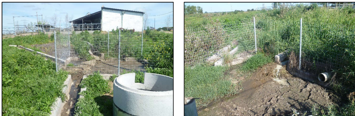
Figures 4-6 Photos of the solids chamber (left: 21/09/2016, right: 03/02/2016)
