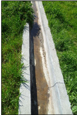
Figures 4-10 Photos of wastewater channels. Left: Concrete open gutter carrying the influent. Right: Excavated-on-soil channel carrying the effluent. (21/09/2016)
