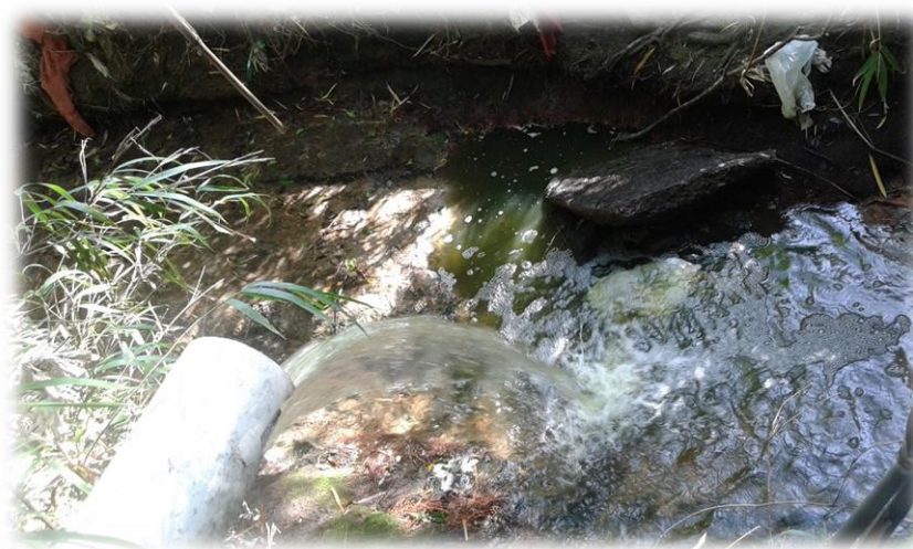
Figure 5: Facultative pond effluent discharge in a small stream that finishes in the Miguelete Creek
