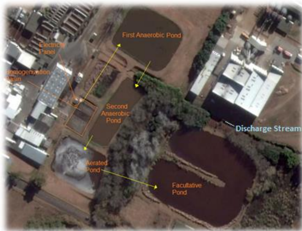
Figure 7: Ponds treatment system for Schneck slaughterhouse
