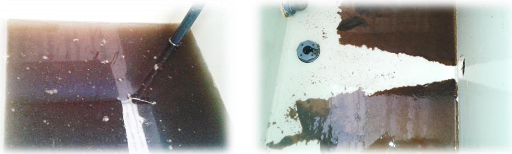
Figure 21: Problem of solids passing to the permeate tank
