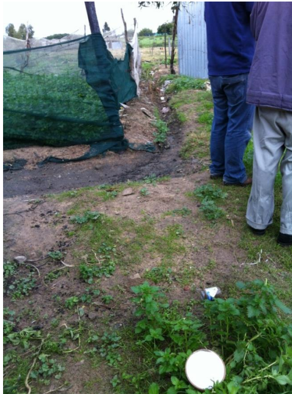
Figure I.2: Septic tank inspection point in Klipheuwel (Pan 18/6/2014)
