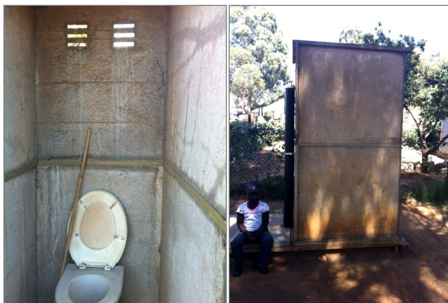
Figure 4.20: Interior and exterior of a well maintained VIP in Finetown (Pan 17/2/2015)
