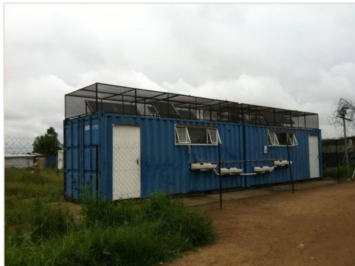
Figure 4.21: Exterior of the Diepsloot pilot CAB (Pan 28/1/2015)
