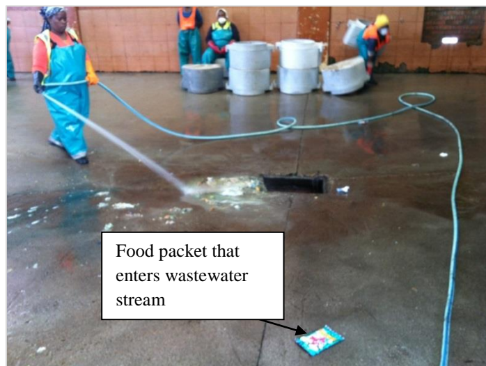
Figure 4.32: Worker hosing contents into faecal sludge disposal point (Pan 23/5/2014)
