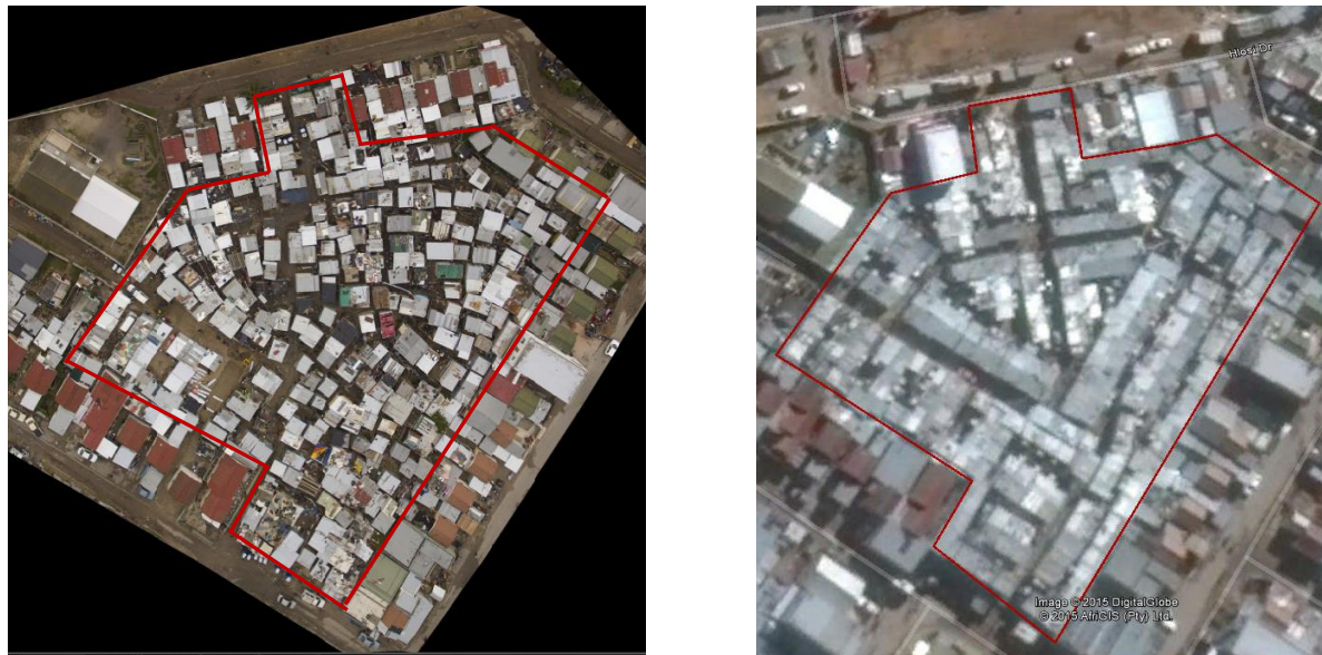
Figure 4.34: Pre- (left) and post-reblocking (right) aerial images of Mtshini Wam informal settlement
