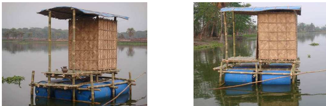
Figure 3.18 Floating emergency latrine [Source: Oxfam]
