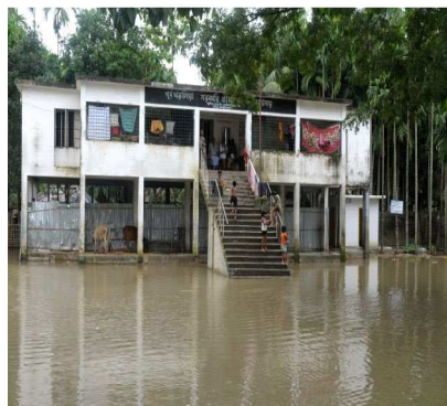
IDPs using the multi-story building toilets [Source: UN News Centre]
