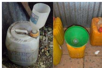
Figure 3.4 Low cost waterless urinal (Source: www.sswm.info )
