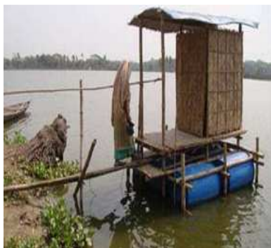
UDL Floating Emergency Latrine [Source: Oxfam]
