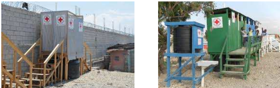
Figure 3.19 Raised toilet units in Haiti [Source: International Federation of Red Cross and Red Crescent Societies]
