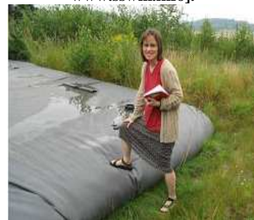
Urine storage tank made of a plastic bladder [Photo commissioned by: E. v. Münch, 2007.]
