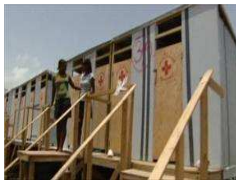
Red Cross toilets in Haiti [source: BBC]
