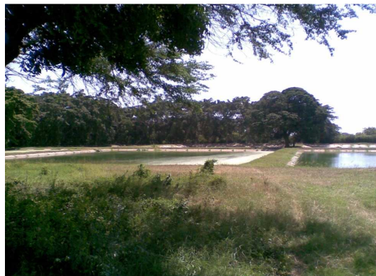
Figure 3.28 Waste stabilisation ponds
