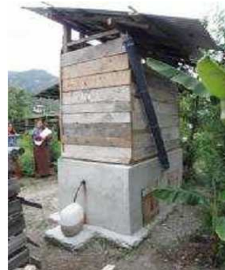
Double-vault UDDT, Vietnamese style, Bhutan [Source: www.sswm.info ].
