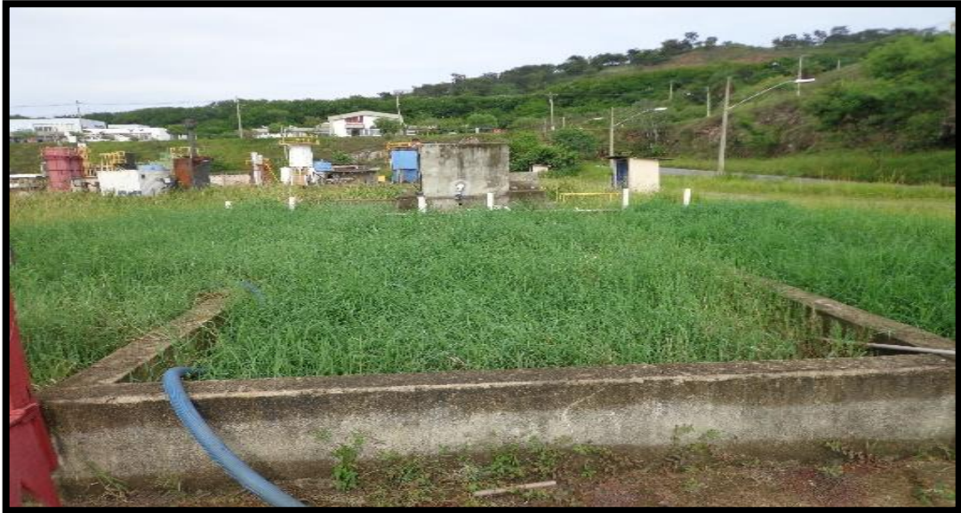
Figure 4.8: Two planted units one in the left and another one in the middle treating domestic wastewater.
