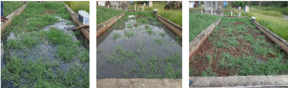
Figure 4.13: Sludge unit being fed by septic tank sludge during operational strategy 2.
