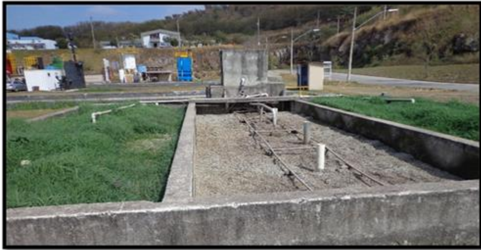
Figure 4.6: Planted unit in the left and unplanted unit in the middle treating raw domestic sewage.
