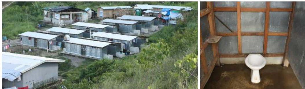
Figure V.11. Latrines at Abucay Bunkhouse (Source: Author, April 2015)
